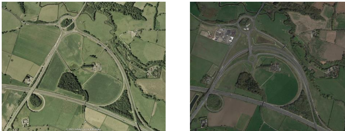
Figure 2 showing aerial images from 2005 and 2021 showing the new road infrastructure associated with the A556/M56 link.
