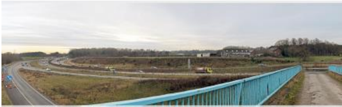
Photograph (2.1 from the Tatton response) – View from footbridge north of Yarwood Heath Farm (Rosthern FP3) Dec 2020 looking south west. The Yarwood Heath Farm buildings can be seen beyond the carriageways and associated bunding and planting.
