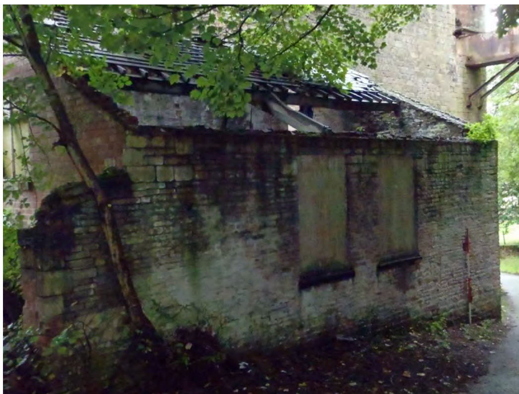
Plate 10: Building G, with shortened northern extent, and blocked apertures in west elevation
