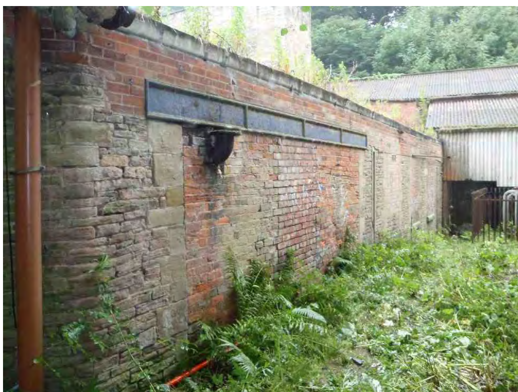
Plate 9: North elevation of Building F, with blocked apertures and rebuilt wall-head
