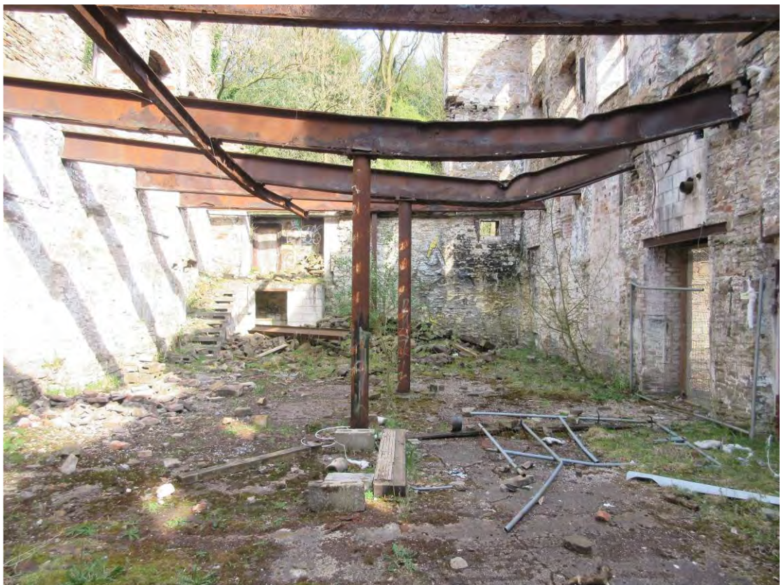
A.12 Damaged First Floor Steel Support Beams
