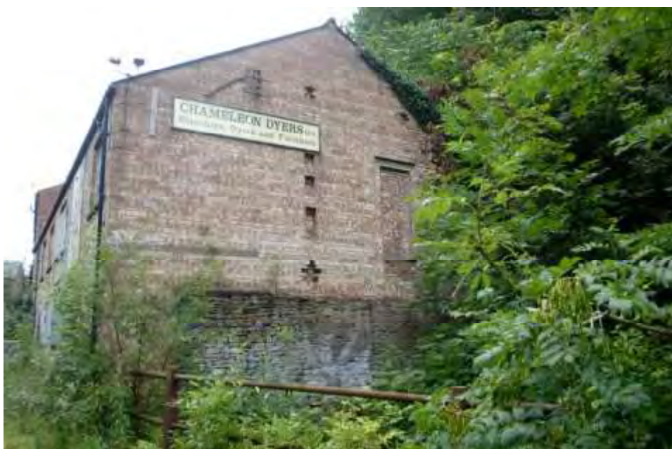
Plate 1: North elevation of Building A, with earlier stone footings at lower level
