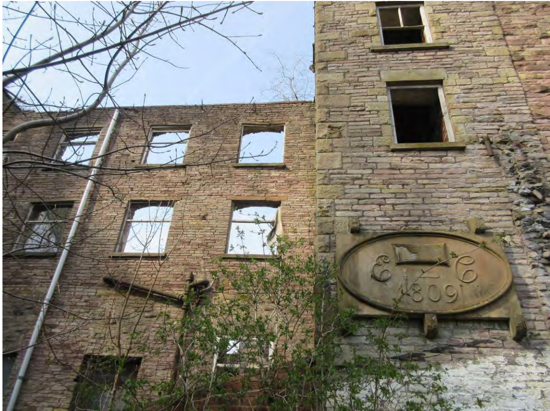
A.5 West Side of South Elevation showing Unstable Stonework
