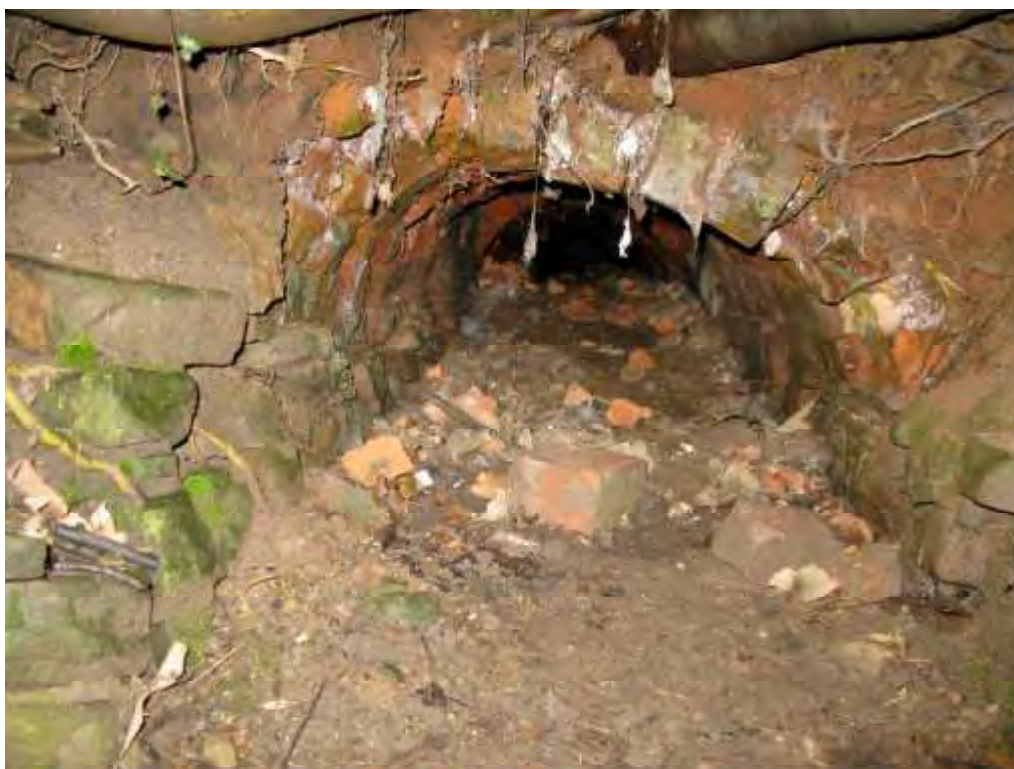
Plate 40: Extant section of flue from boilers within Building E to demolished chimney above
