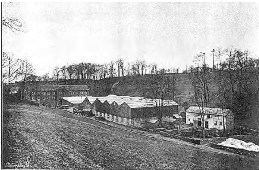
Fig 9: the buildings at Ingersley Vale as seen from the south in 1900 showing the small finishing shed, the large finishing shed and warehouse built in 1896 and the white cloth store room, making-up, stamping and packing room and stables (extreme right) built in 1899.
