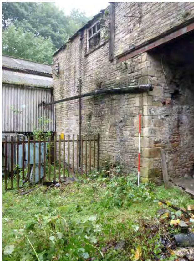
Plate 5: South wall of western part of Building E, with arched aperture to west of entrance
