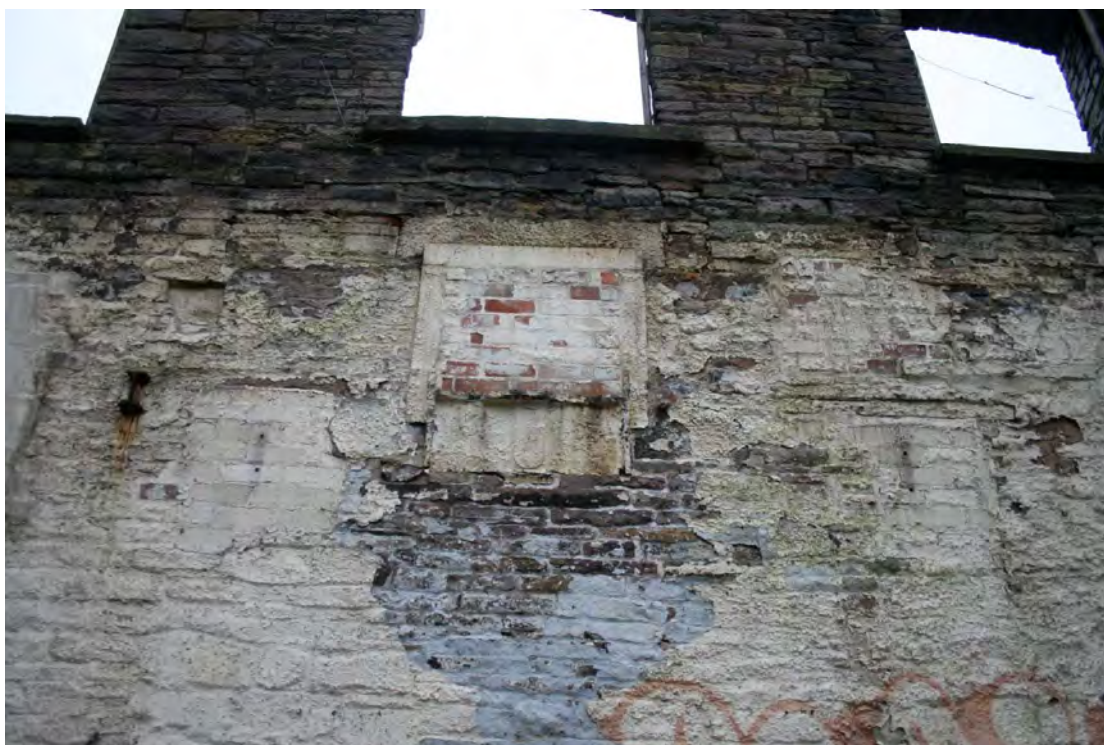
Plate 19: Large cast-iron bearing box, Bay 7, Building I, flanked by smaller apertures
