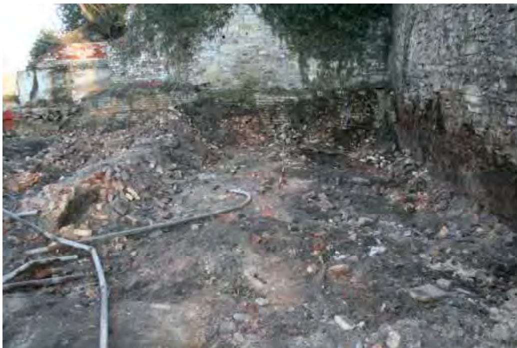
Plate 35: Footprint of Building E following demolition
