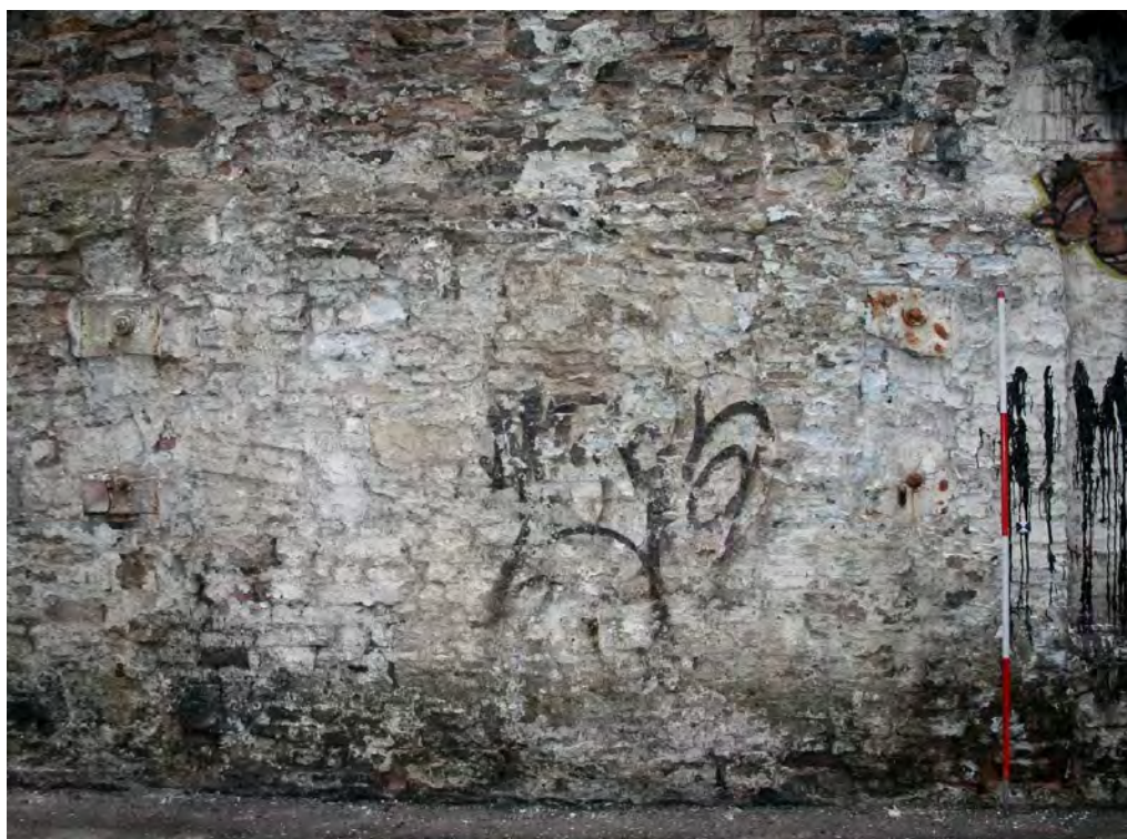
Plate 23: Broken cast-iron wall brackets, north elevation, Building I
