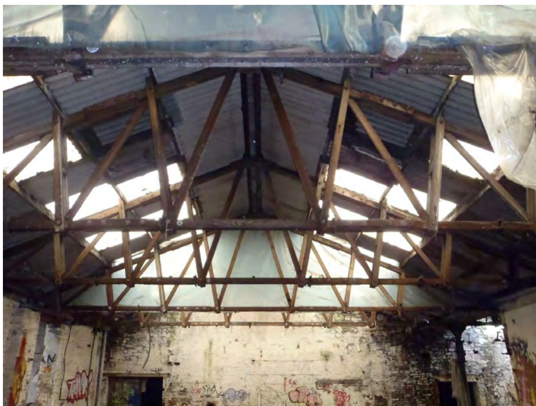
Plate 15: Rooftrusses within Building Q,
