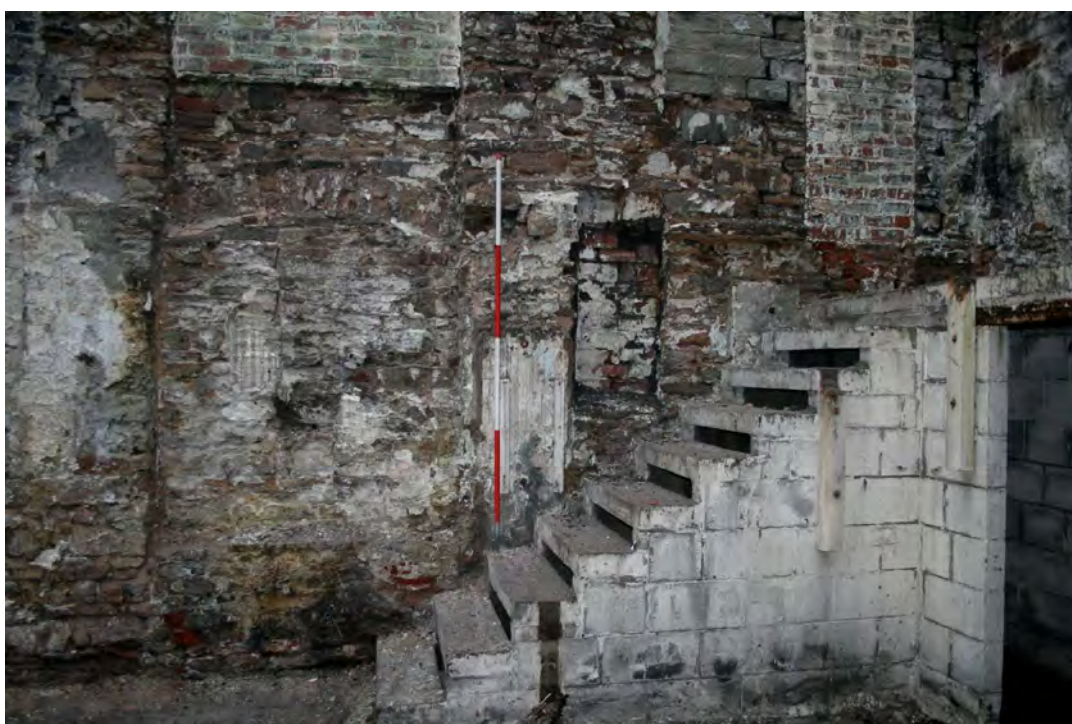
Plate 25: Blocked windows, inserted stair, and possible blocked end bearing bracket, Bay 12
