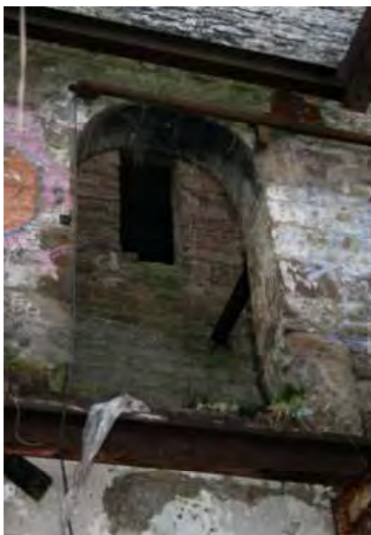
Plate 22: Detail of axle mount for water wheel, with cut padstone
