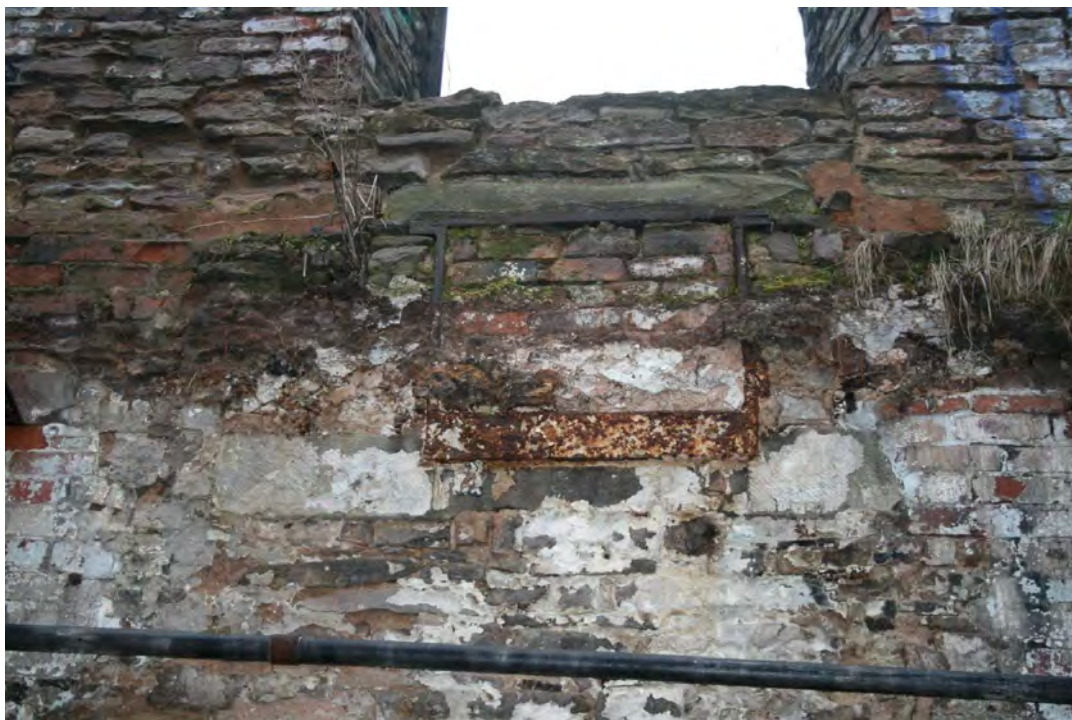
Plate 24: Large cast-iron bearing box, Bay 7, Building I, flanked by smaller apertures
