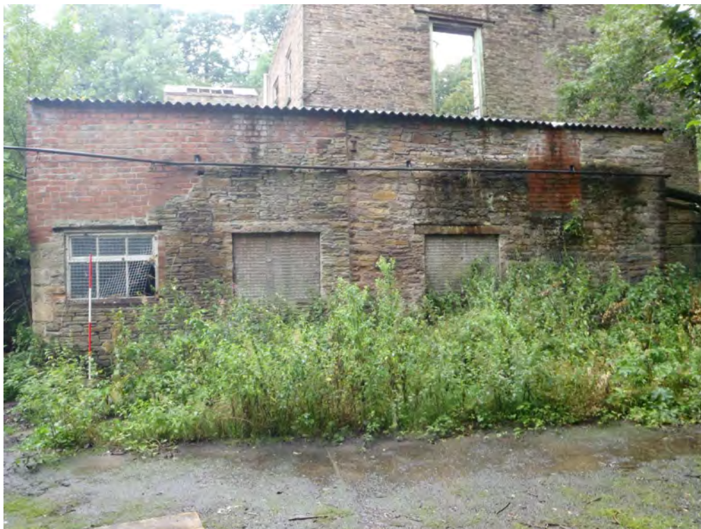
Plate 12: East elevation of Building L, with central butt-joint within stone construction
