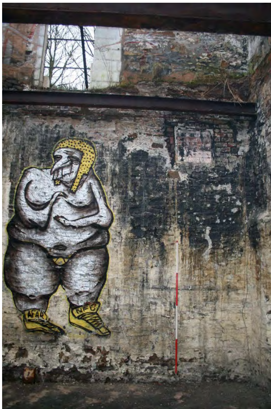
Plate 26: Blocked end bearing box, eastern gable, Building I, with remodelled doorway above
