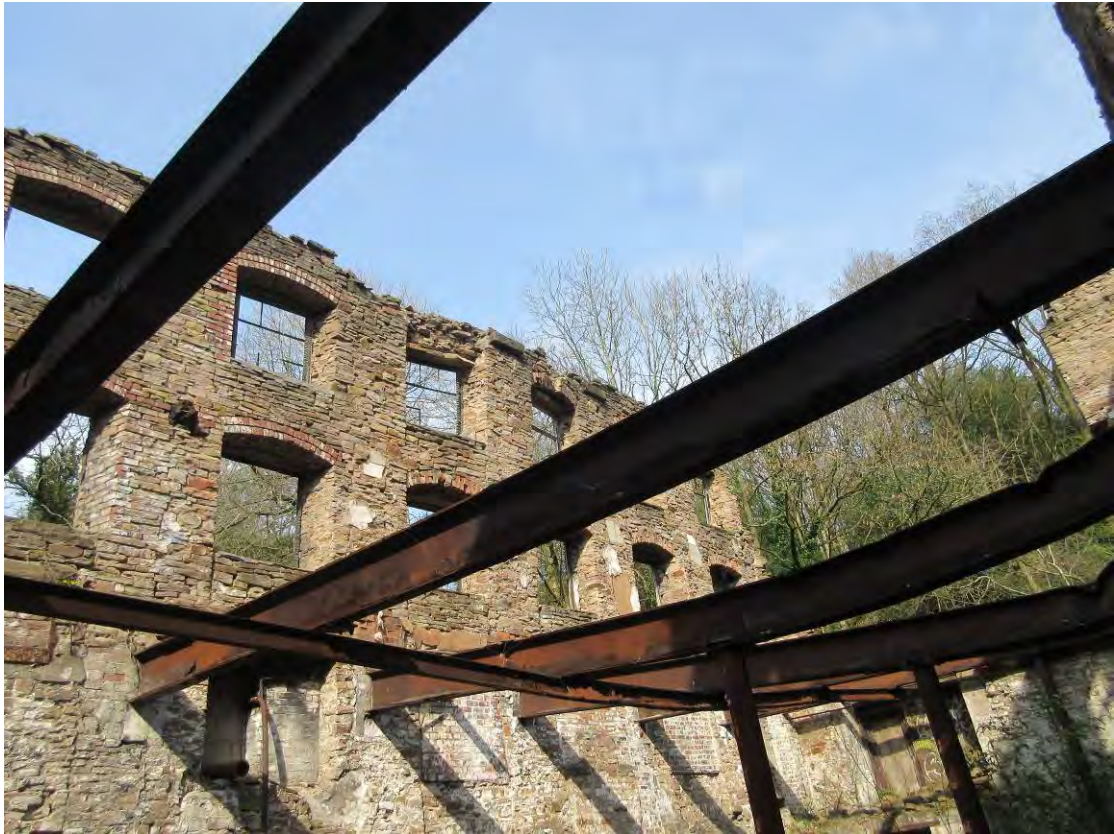
A.13 Movement and Damage to North Elevation Wall
