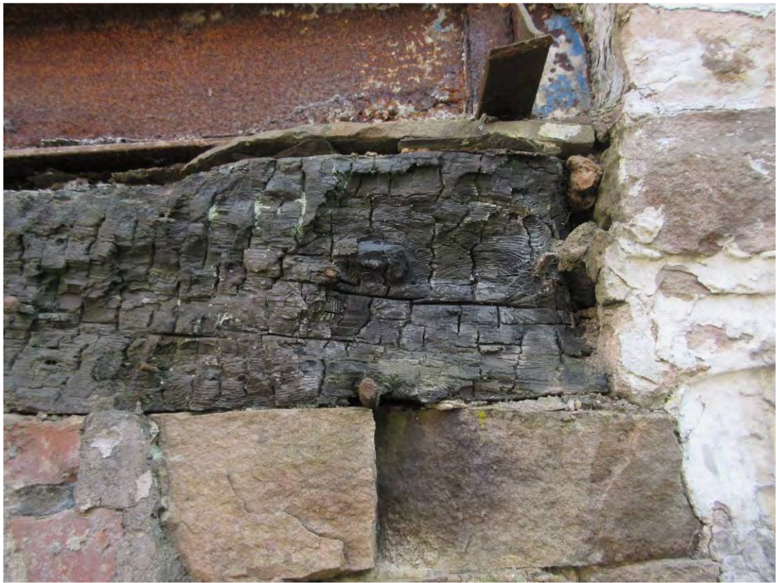
A.14 Fire Damaged Timber Built Into South Elevation Wall
