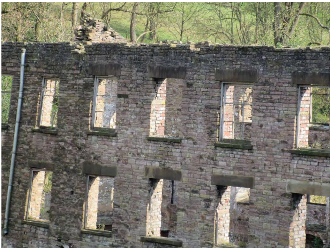
A.10 Damage to Head of North Elevation Wall
