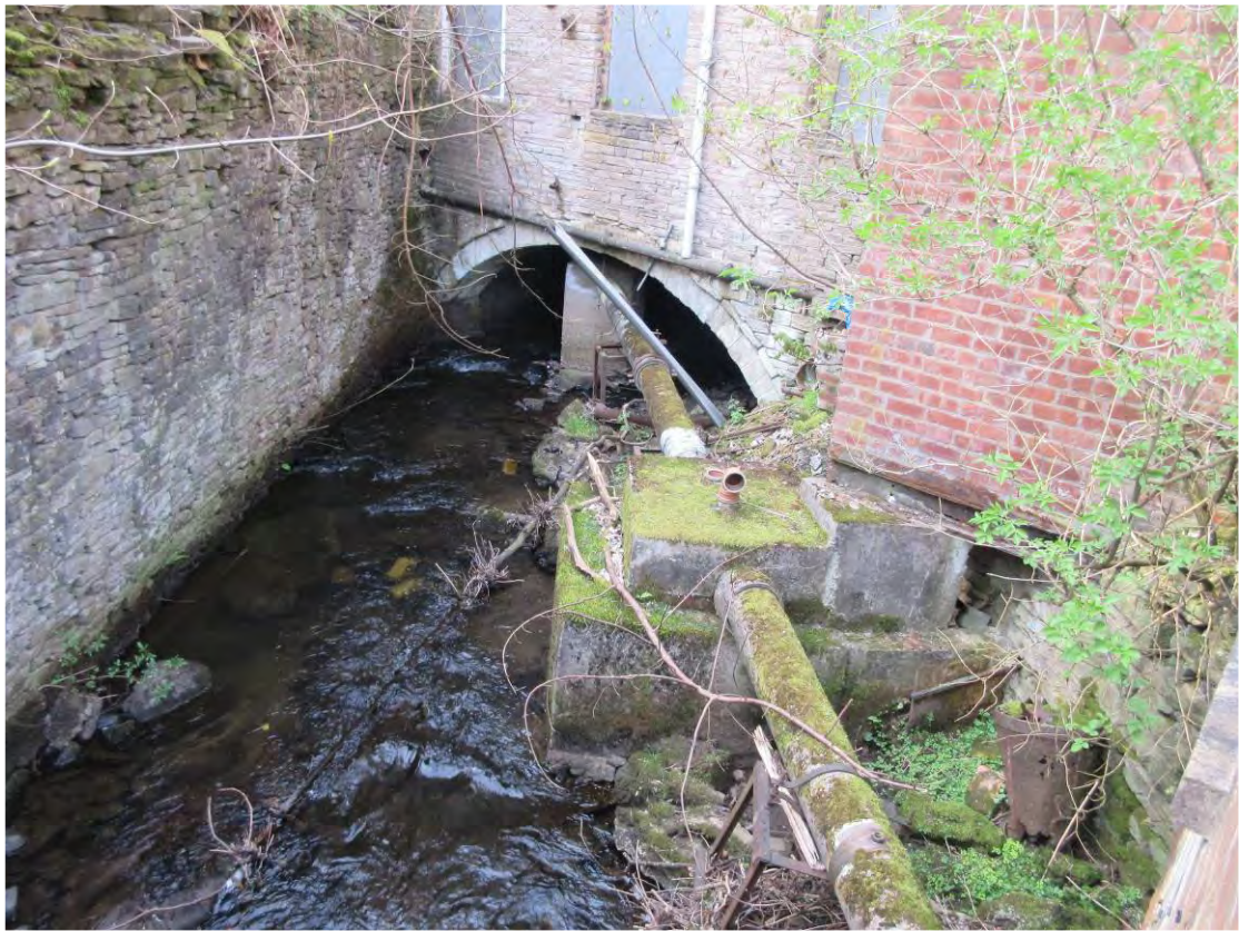
A.4 Masonry Arch Supporting West Side of South Elevation
