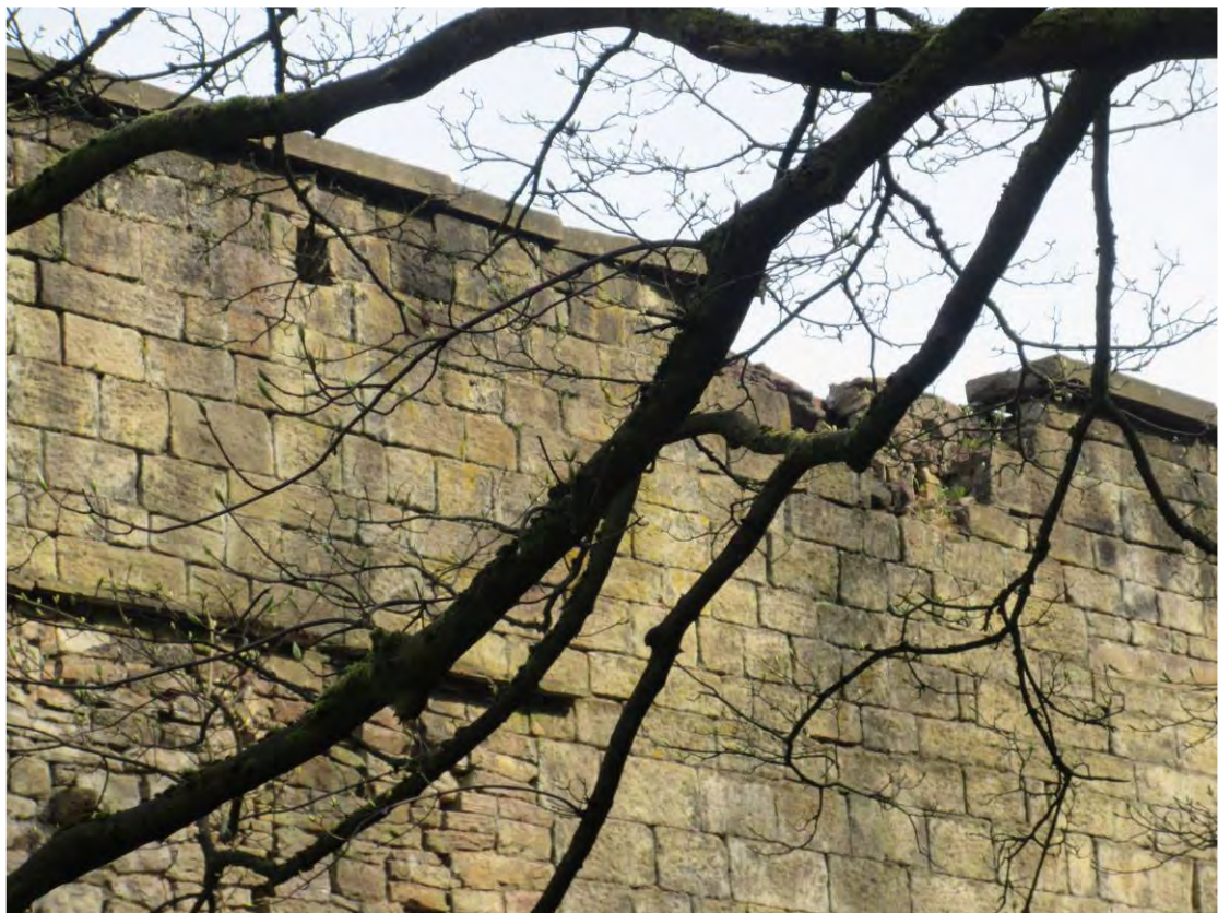
A.8 Local Damage to Parapet of Wheel House
