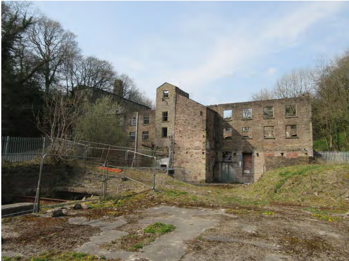
A.1 South Elevation of Building
