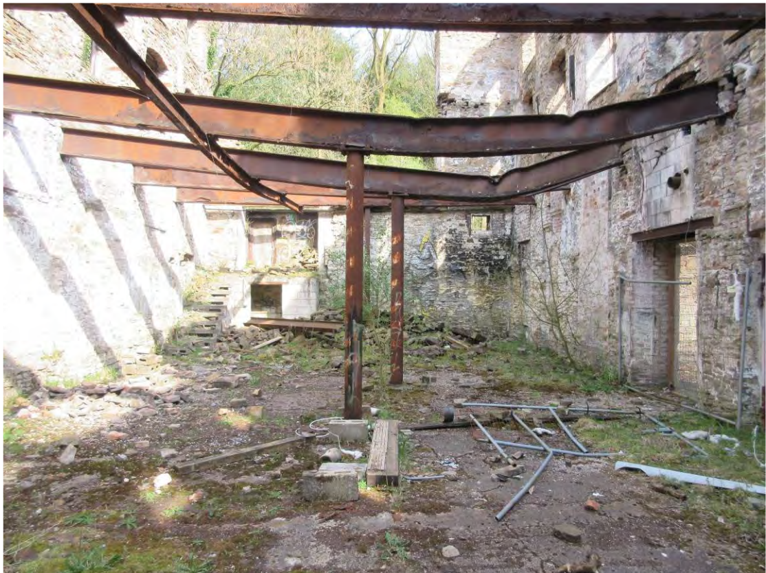
A.12 Damaged First Floor Steel Support Beams
