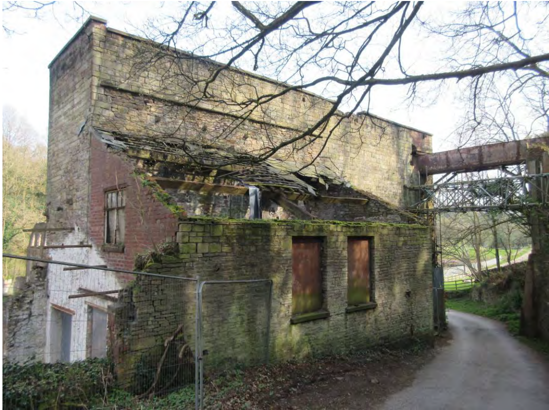
A.7 West Elevation of Wheel House Showing Aqueduct
