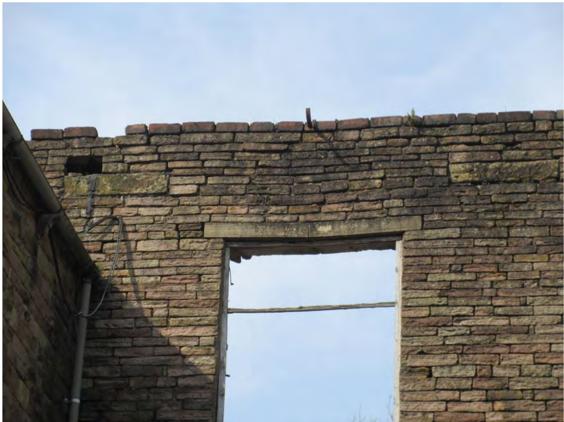
A.2 Fractured Lintel and Unstable Stonework
